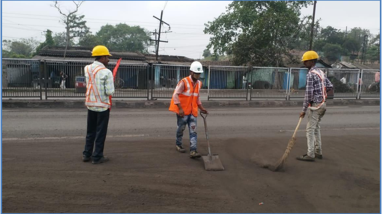
Picture 3 – Road Cleaning (Mechanical Sweeper and Manual Sweeping)
